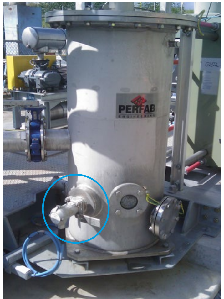
Trimod'Besta level switch for low level alarm
