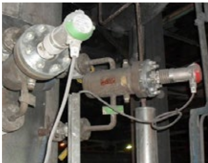
Level switch type: HAA 22C01 041 with float chamber: I021-1C0RC1
